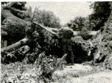
R.R. clearing trees for the parking lot expansion.
